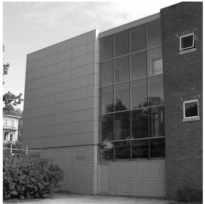
The glassed-in link connects The Cube (on the left) with the original 1916 building, containing offices and the cinema. This transitional space, a route from the parking lot, is kept at a moderate temperature.
